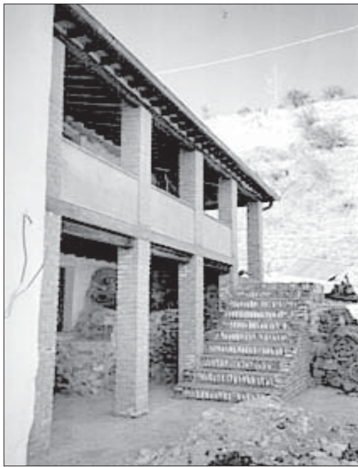
Serkhang under construction
