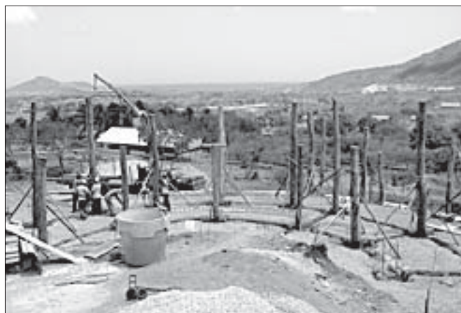
Setting the poles for Rinpoche's house
